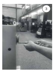
Secure the duct with the 4 screws provided and a screwdriver.
