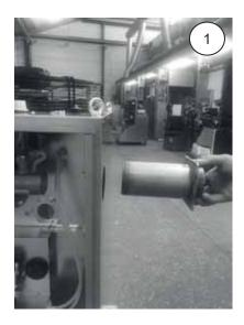
Insert the air duct into the hole provided for this purpose on the upper side of the appliance.
